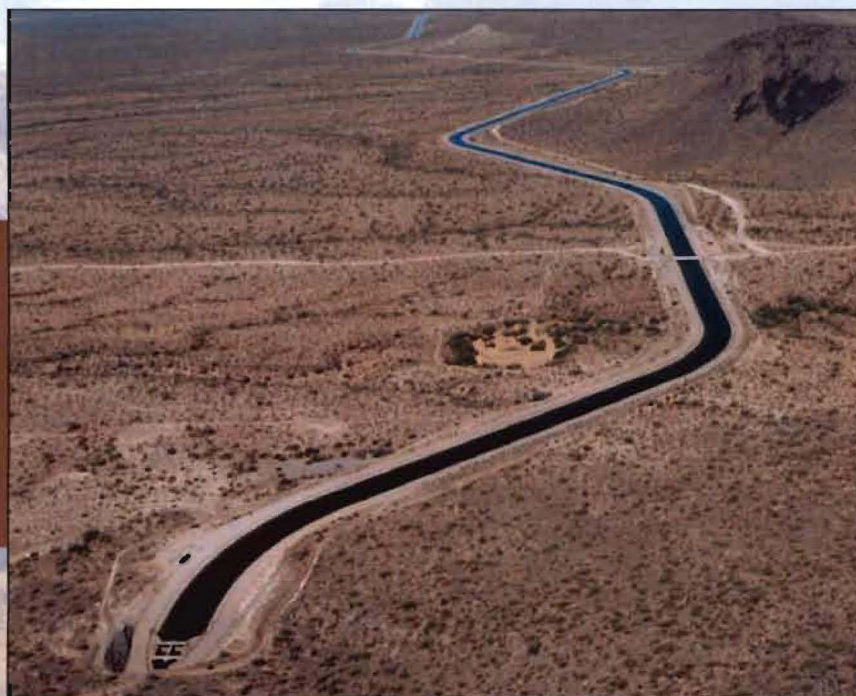
Central Arizona Project transports water from Lake Havasu, which straddles the border between Arizona and California, across the desert via a 366-mile-long water conveyance system.
