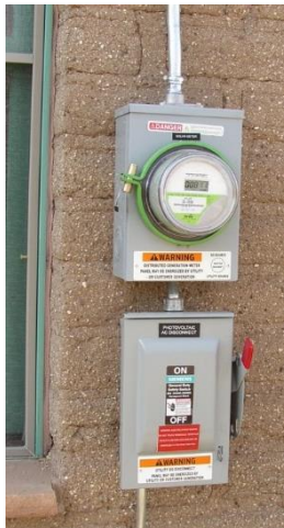
Net Meter & Electric Panel
